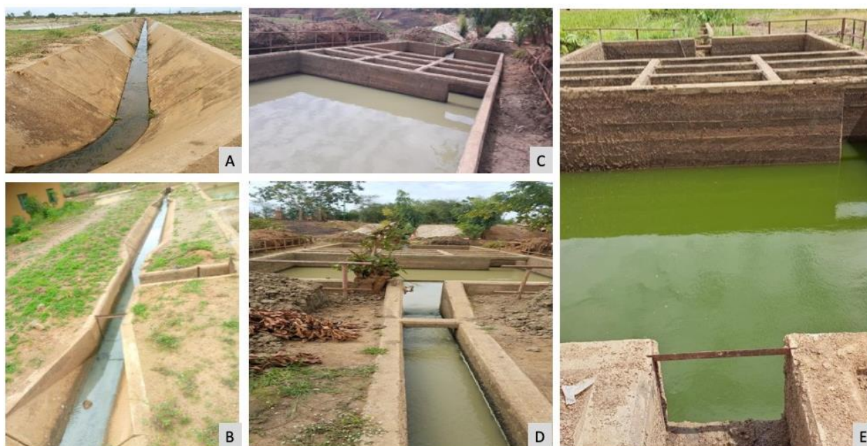
Figure 10. A model of an aquaculture water purification system. The decantation water treatment systems (C, D and E) with the main discharge and drainage channels (A and B) to the wastewater treatment plant. All wastewater from the hatchery, tanks and ponds is discharged through a drainage channel to the decanting device where it is treated and then reclaimed by the local farmers for vegetable cultivation, fruit cultivation, etc.
