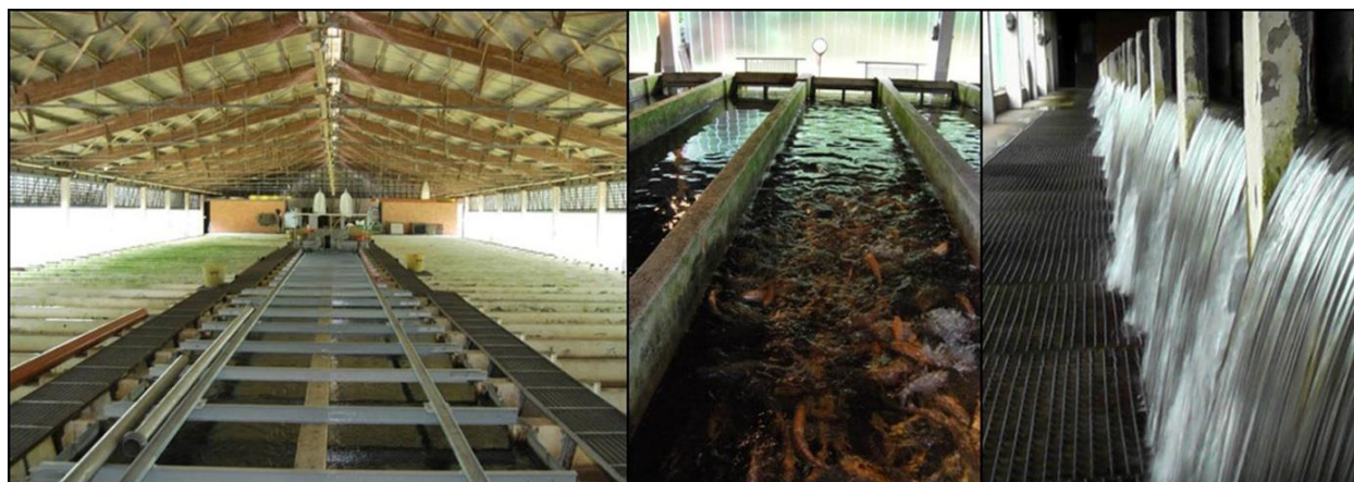
Figure 1. Picture of the flow-through aquaculture system Forellezucht Uhthoff, Neubrandenburg, Germany (Clois-Fuentes et al., 2024). The overview of the facility with the inflow (left), a closer view of the concrete raceways (middle) and an image of the water discharging from the raceway tanks (right).
